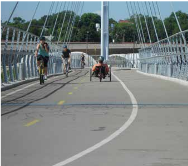
Martin Olav Sabo Bridge, Midtown Greenway: Minneapolis
