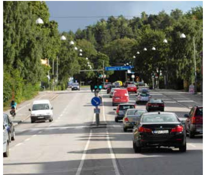
Where roads are difficult to cross - as here in Stockholm - bi-directional tracks on each side respond to natural demand
