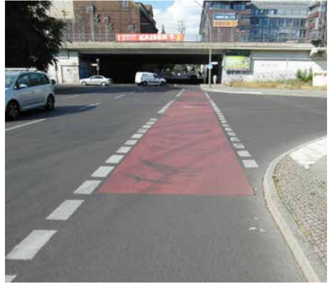
Berlin - coloured surfacing used to emphasise the cycle lane as it crosses a side street
