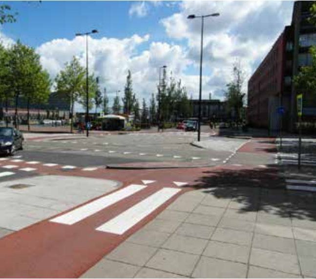
Amsterdam - a simple priority crossroads with parallel cycle and pedestrian crossings (with 'sharks' teeth) on all arms
