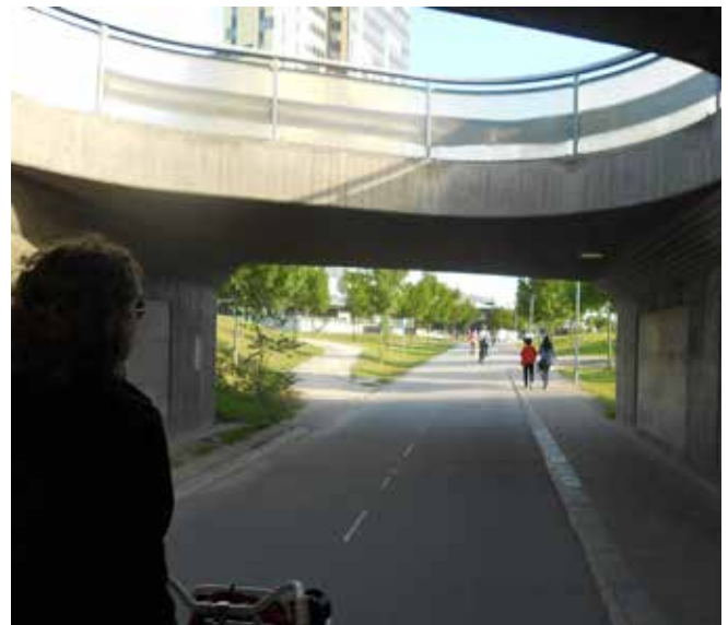
Separate, parallel cycle and pedestrian paths beneath a major traffic junction: Lund
