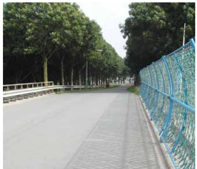
The same bridge over the A27 has a custom-designed metal lattice screen on one side to act as a wind break
