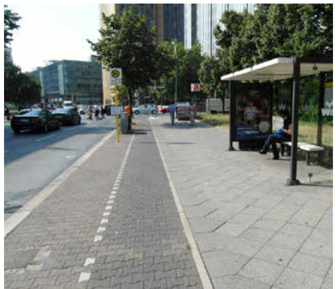
Berlin - an off-carriageway cycle track passing in front of a bus stop
