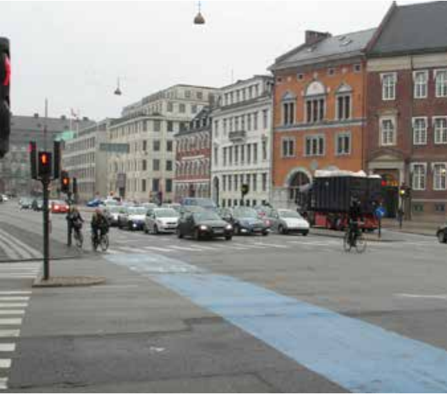
Copenhagen - unbounded cycle lane markings through a busy junction
