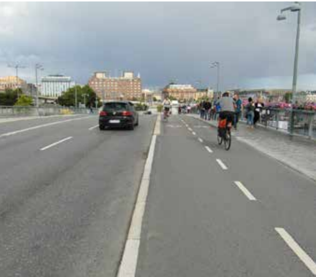
One of several bridges in Stockholm where a former traffic lane has been re-used as a bi-directional track
