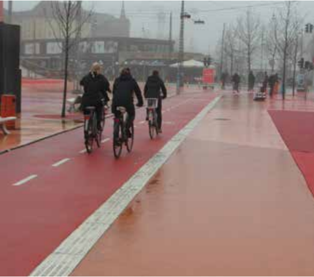
A bi-directional track runs through the one-of-a-kind urban realm of Superkilen in Copenhagen
