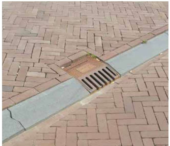
Houten: a 'forgiving' kerb at the edge of a cycle track - angled to avoid being clipped by pedals on the down-stroke
