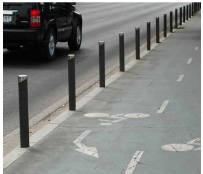
Seville - non-flexible wand-like bollards
