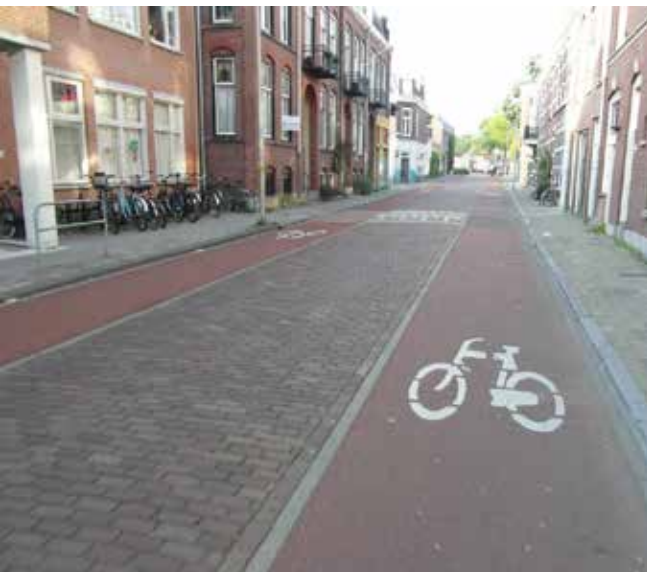
Utrecht - dark red coloured asphalt is the default material for cycle tracks
