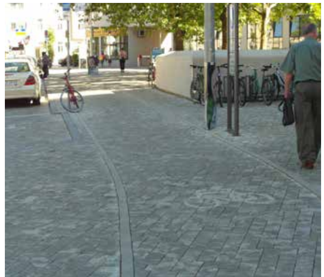
New public space at Am Harras, Munich: parking bays, cycle path & footway in same materials with small step separation
