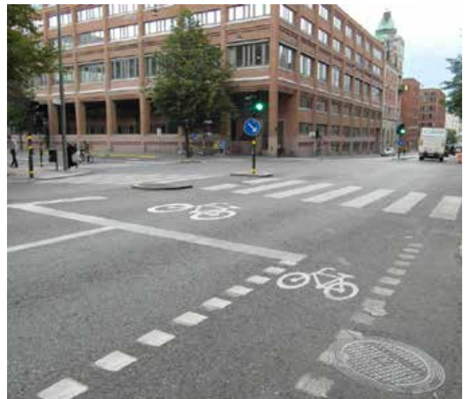
Another full-width ASZ, in Stockholm. These are uncommon because two-stage left turns are the norm.
