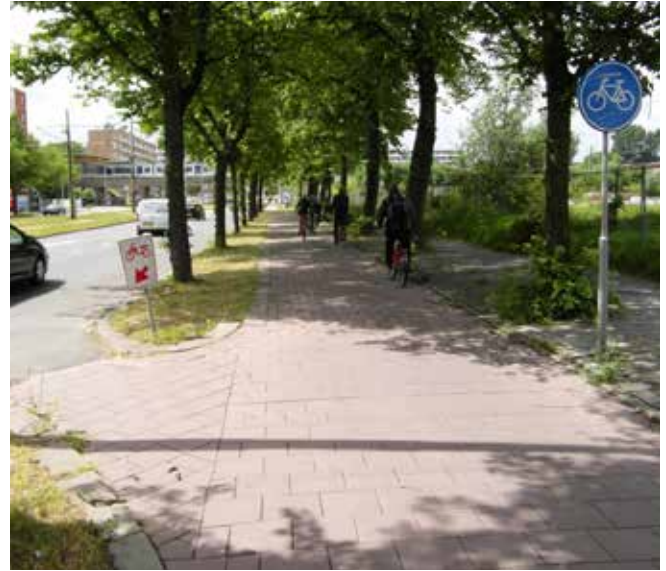
...but not when signs clearly state they should use the main carriageway
