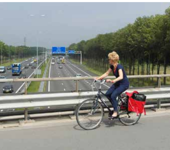
Low-parapet cycle, pedestrian and local access-only bridge over the A27 motorway between Utrecht and Houten
