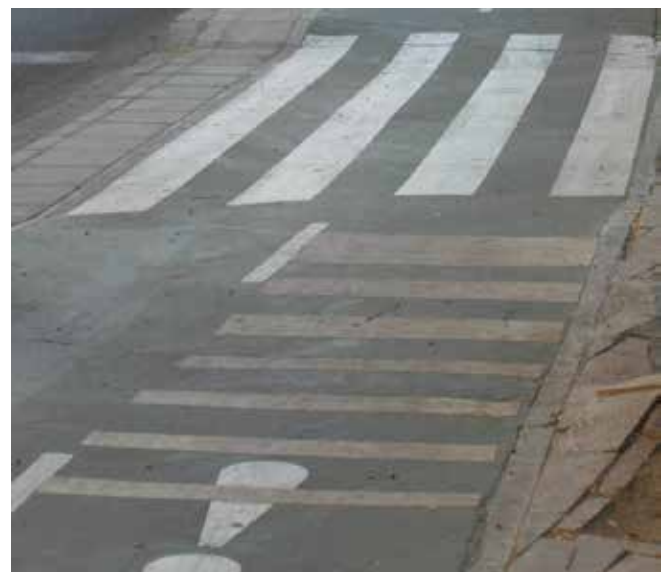
Seville - typical warning to cyclists on approach to a pedestrian crossing
