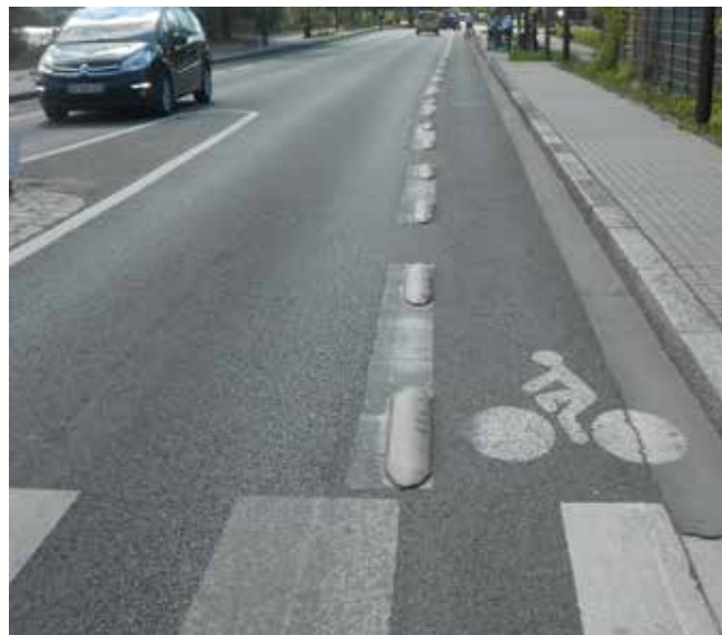
Raised thermoplastic markings: Nantes
