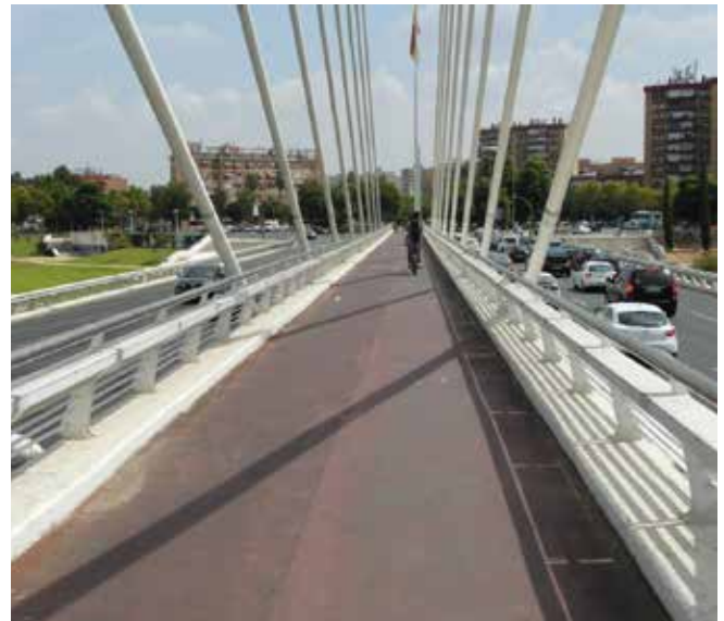
Seville - Puente del Alamillo, with a central pedestrian-cycle path integral to the design
