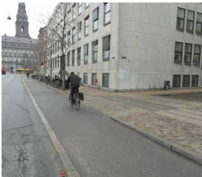
Copenhagen - no break, markings or other differentiation as this cycle track crosses a minor side street
