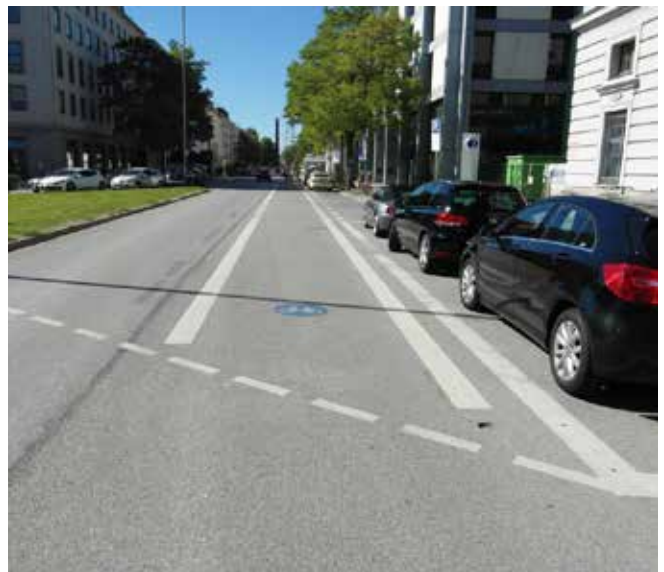
Munich - a well-proportioned cycle lane, plus buffer, where previously there was a second general traffic lane
