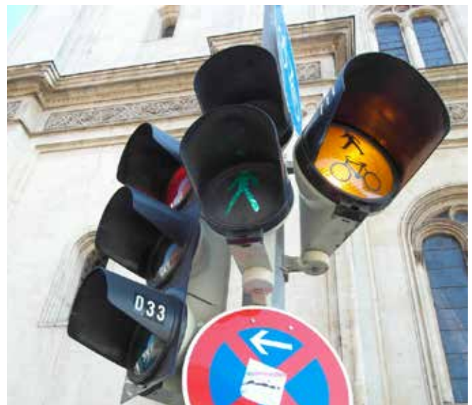
Munich - here, the flashing amber indicates that drivers must give way to cyclists and pedestrians when making a left turn
