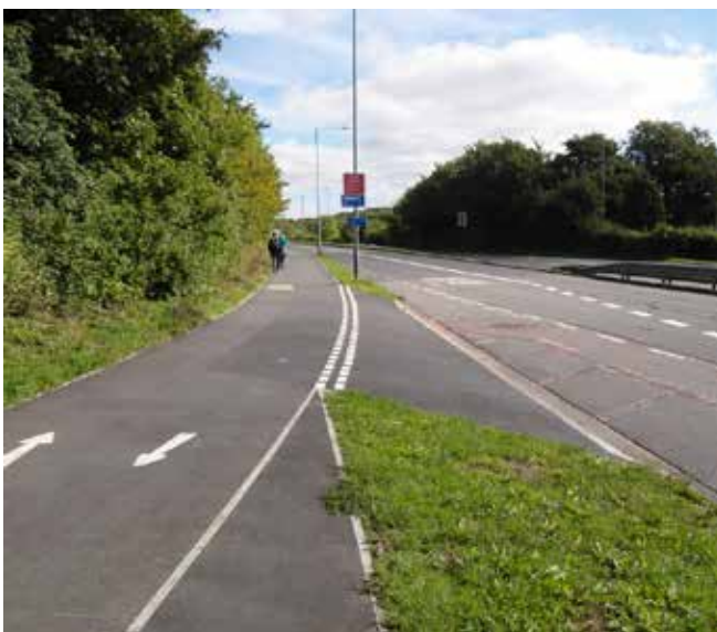
Brighton & Hove - a gentle transition from on-carriageway cycle lane (in bus lane) to off-carriageway 'shared use' path
