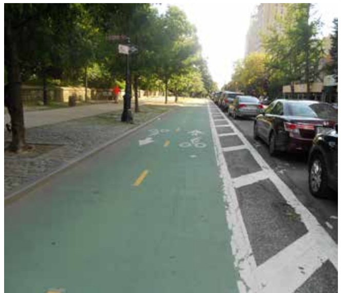
A bi-directional track in Brooklyn, lightly-segregated by a wide painted buffer strip
