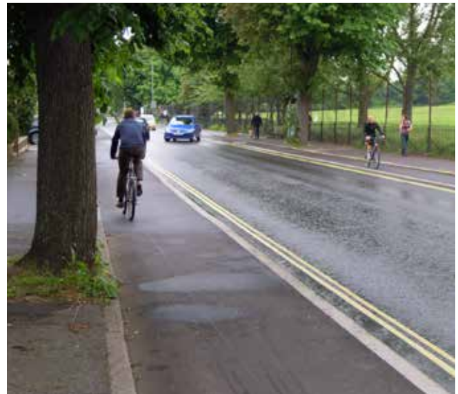
Old Shoreham Road in Brighton & Hove: a 6.1m carriageway with no centre-line between stepped cycle tracks
