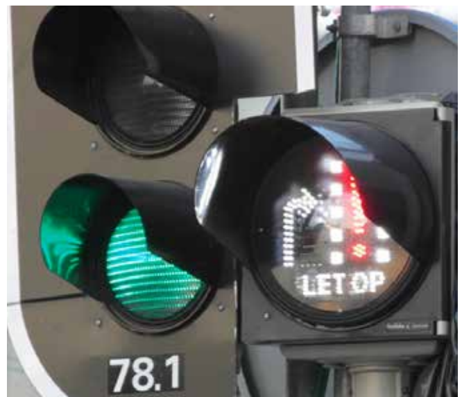
Utrecht - informative signal aspect cautioning right-turning drivers to watch for crossing cyclists and pedestrians
