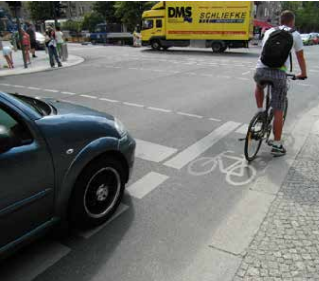
A very short nearside lane ASL in Berlin - does the minimum of putting the cyclist plainly in a car driver's line of sight
