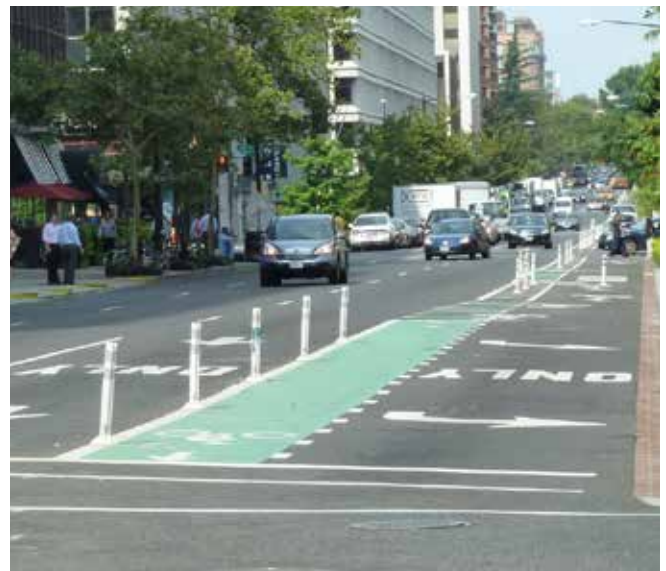
Washington DC - a similar arrangement to the Berlin example, but with 'wands' used to limit the crossing section
