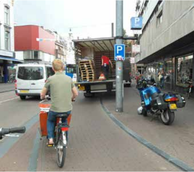
Utrecht - stepped separation provides good protection, but is not an uncrossable barrier to vehicles
