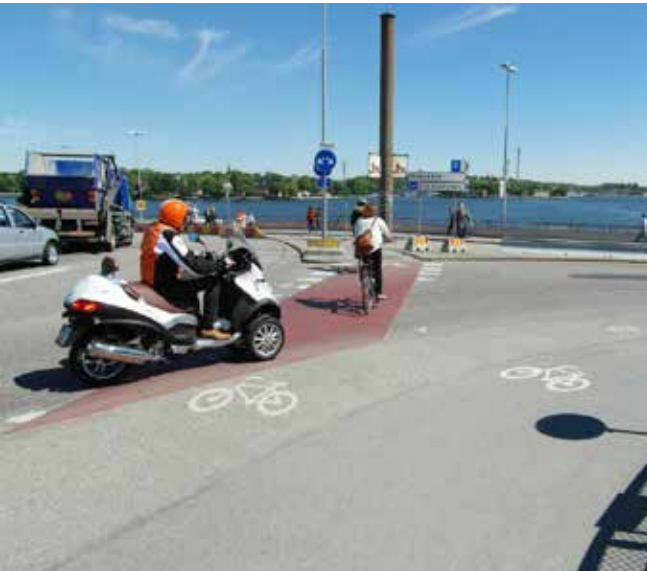
Stockholm - coloured surfacing used to highlight a cycle lane, as it crosses the exit arm of a major junction
