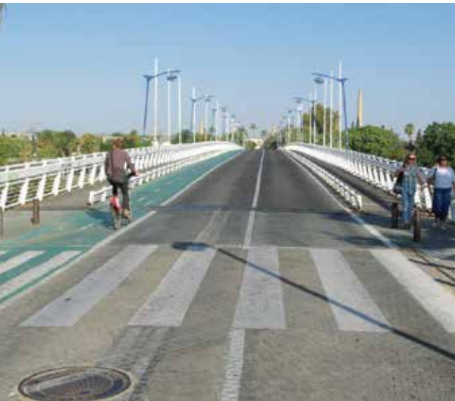
Seville - the Puente de la Cartuja, though narrow, had part of the carriageway reassigned to cycles in the mid-late 2000s
