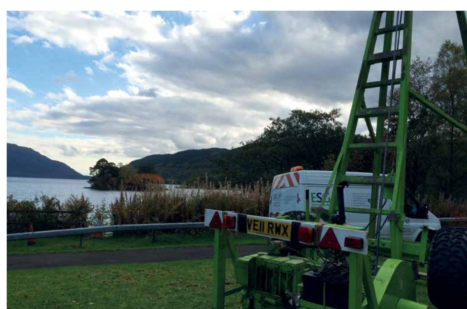
Preliminary ground investigation work.
