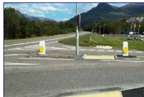
Figure 7.9: Crossing of side road using central islands with vehicle priority
