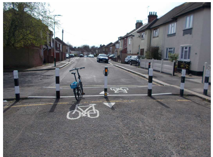
Queens Park Road, Romford. Lockable bollard (centre).
