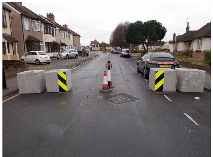
Cedar Road, Romford. Experimental closure to motor traffic using Legato [7] concrete blocks, and a removal bollard with a fire brigade padlock.
