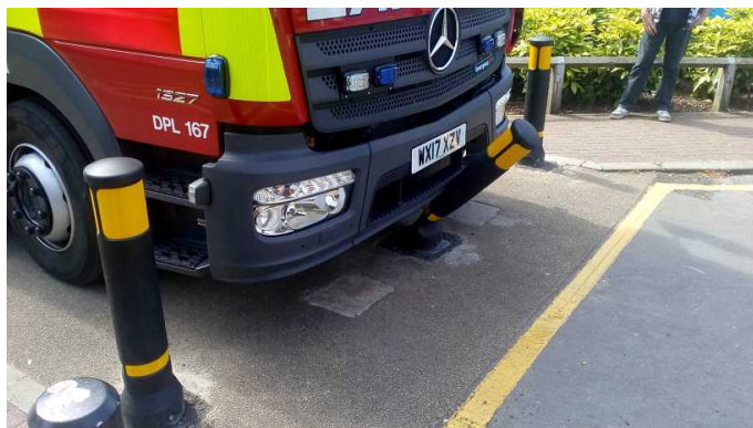
Park End Road, Romford. Collapsible bollard.
