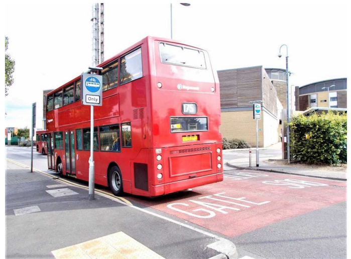
Oldchurch Rise, Romford. Traffic signed bus gate with fixed CCTV enforcement cameras.
