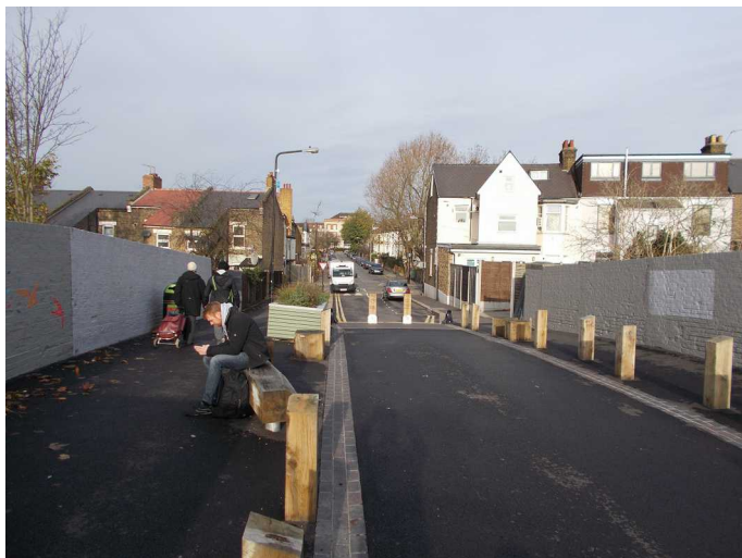
West Avenue, Walthamstow. This railway bridge is essentially a large modal filter which was closed to motor traffic because of structural issues. It's now a place to sit and think as well as walk and cycle through.
