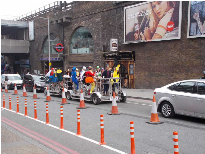
Tooley Street, Borough. Temporary contraflow cycle lane, protected with traffic cylinders.
