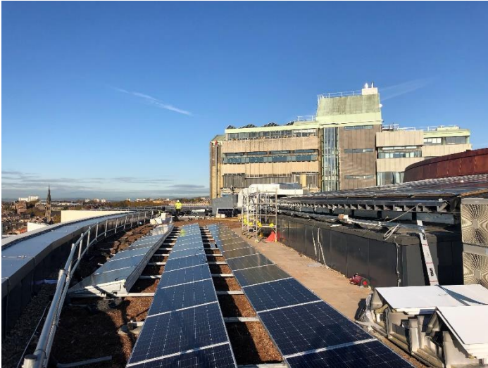
Solar Panel installation on the James McCune Smith Learning Hub roof
