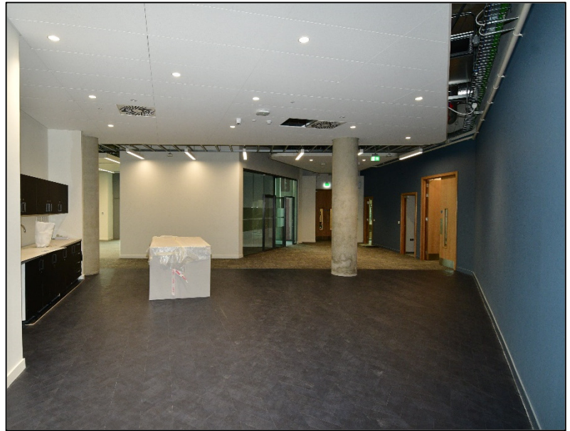
Interior progression – Advanced Research Centre – Level 3
