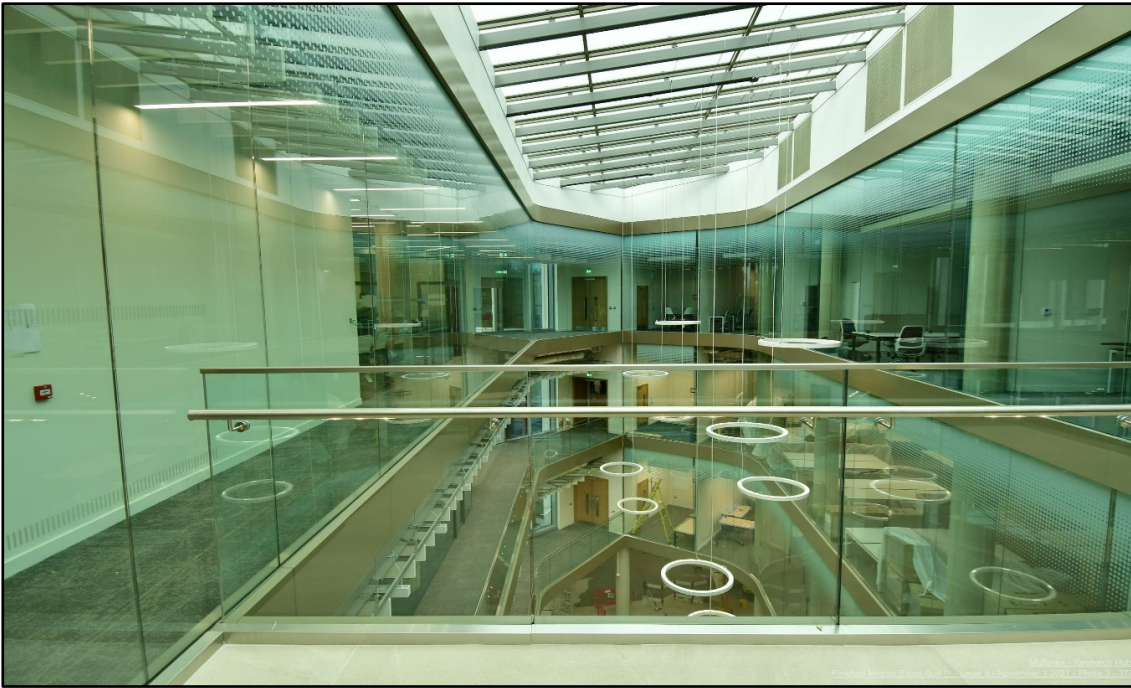
Interior progression – Advanced Research Centre – Atrium
